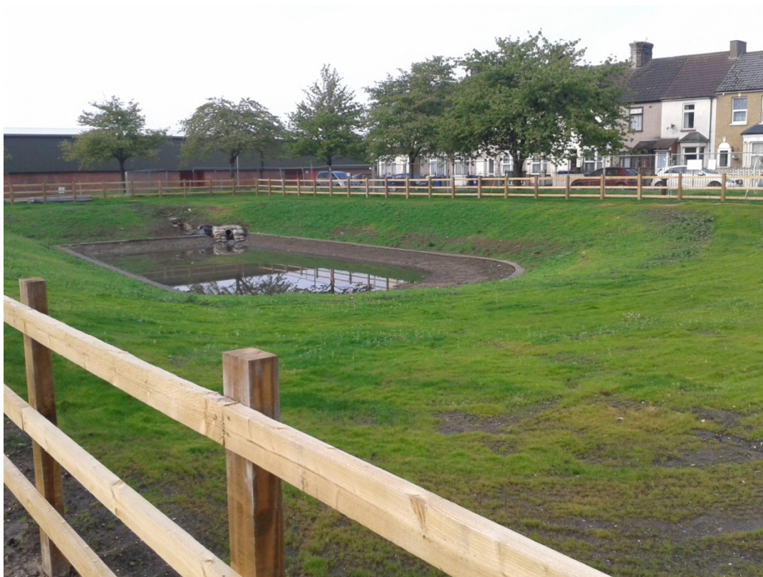
Figure 1: Drainage Pond at Gumley Road
